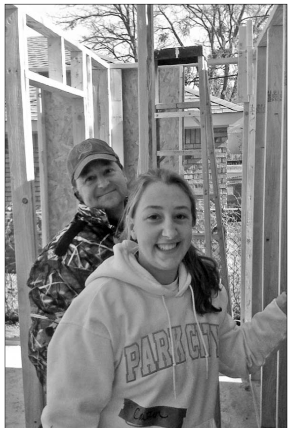
Brett and Caitlin Smith work together during the build.
